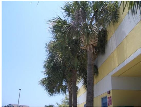
Fig 1. Palm trees contacting a structure.
