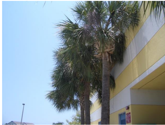
Fig 1. Palm trees contacting a structure.
