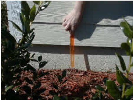
Fig. 1. The current building code requires at least a 6 inch inspection gap, as shown in the picture above. The inspection gap between mulch and siding on the home will allow anyone to see if termites are building mud tubes into a structure.
