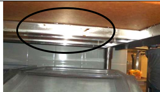
Figure 7. Area under kitchen counter where heat from the nearby stove has melted the bait. Note that the bait has dripped down to the edge of the frame.
